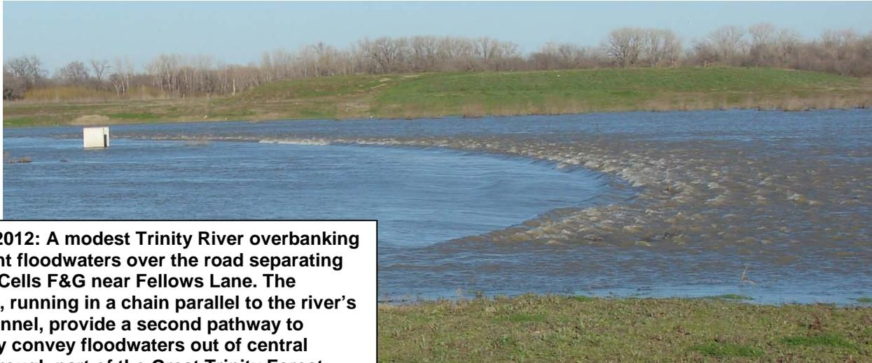
**Jan. 27, 2012: A modest Trinity River overbanking event sent floodwaters over the road separating Wetland Cells F&G near Fellows Lane. The wetlands, running in a chain parallel to the river's main channel, provide a second pathway to efficiently convey floodwaters out of central Dallas through part of the Great Trinity Forest before rejoining the main channel near Great Trinity Forest Way (Loop 12) in southeast Dallas.**
